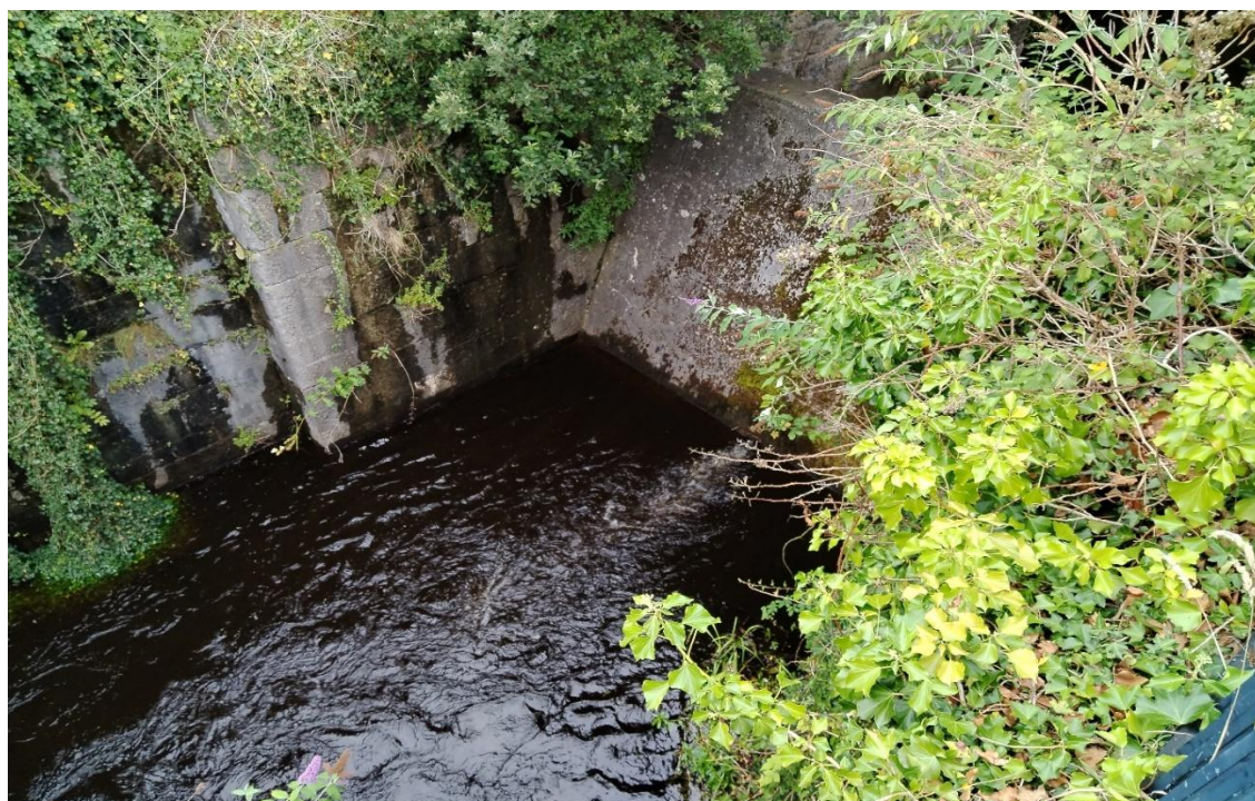
Figure 4. Fast flowing waters exiting the sluice.
